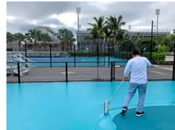
Applying the LM Topcoat
