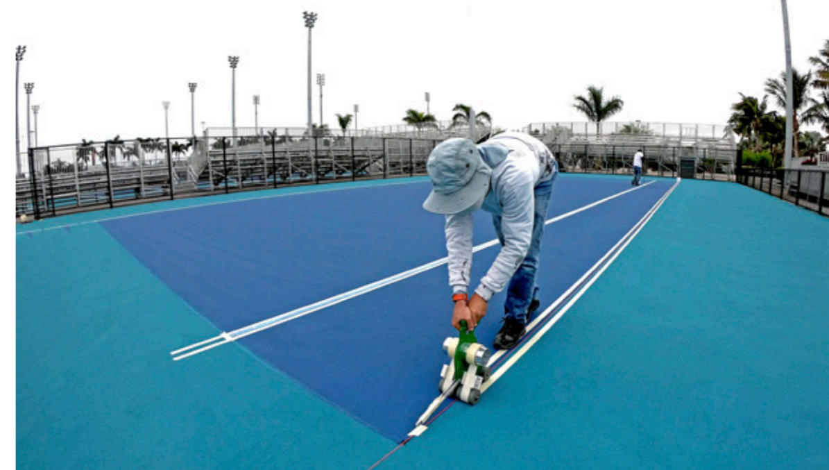
Taping in preparation for line paint
